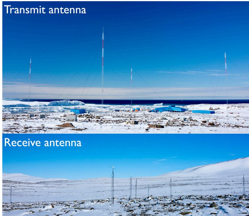
**Fig. 3.** Photos of the JBS-VIPiR antenna system. Four 36-m towers for the transmitting antenna and 76-m towers for the receiving antenna are displayed. JBS-VIPiR, Jang Bogo station-vertical incidence pulsed ionospheric radar.
